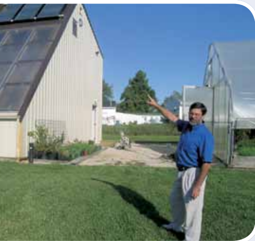
Barry Adler's bio-integrated greenhouse in Plain City, OH is powered by a wind turbine and solar array, and heated by a solar thermal, drain-back, closed-loop radiant floor system. Photo by Joan Benjamin.
